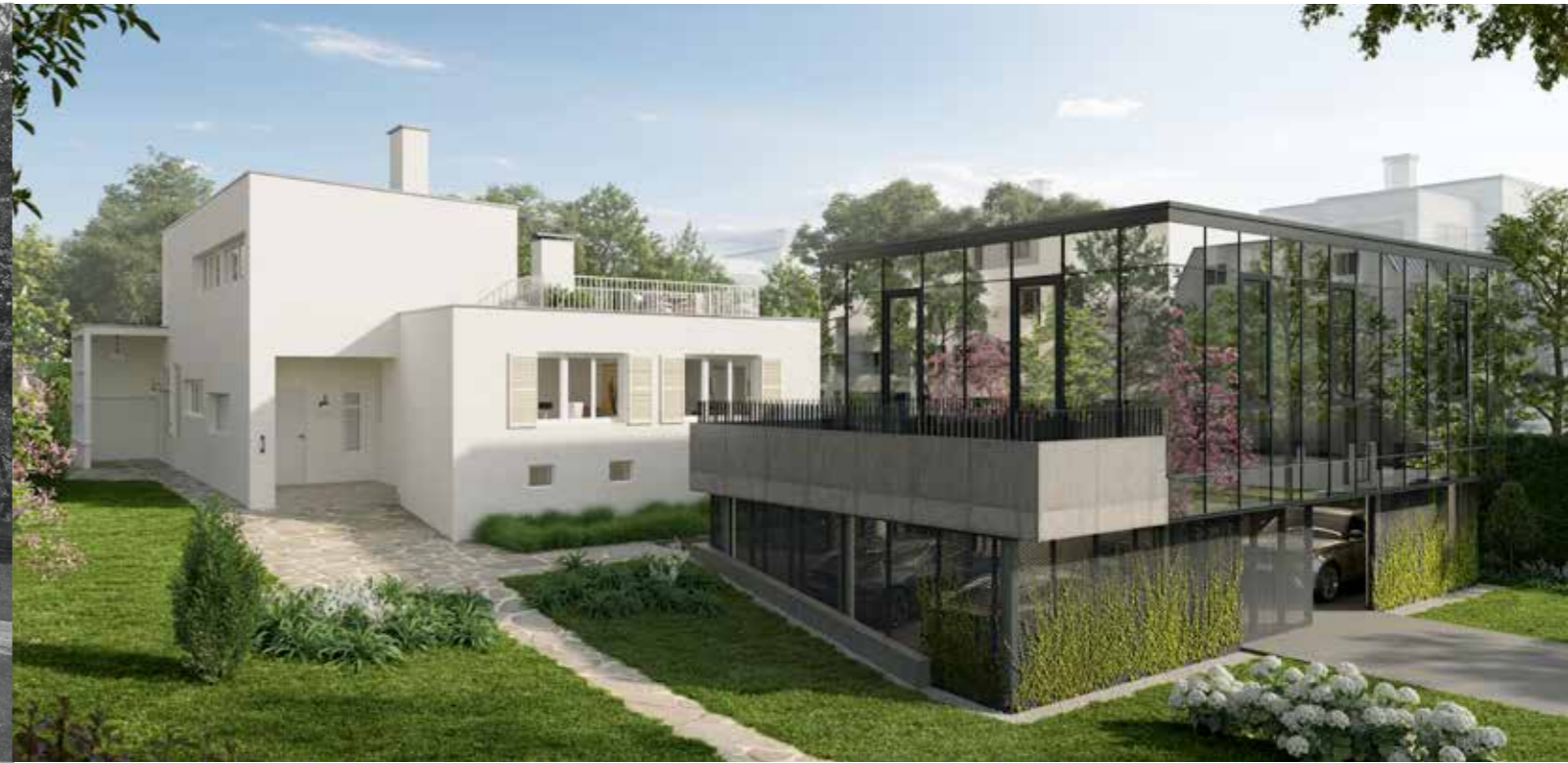
Almost 90 years after the building was completed, today Villa Bunzl has been returned to its former splendour – augmented by a structure positioned before the house that creates space for new ideas.
